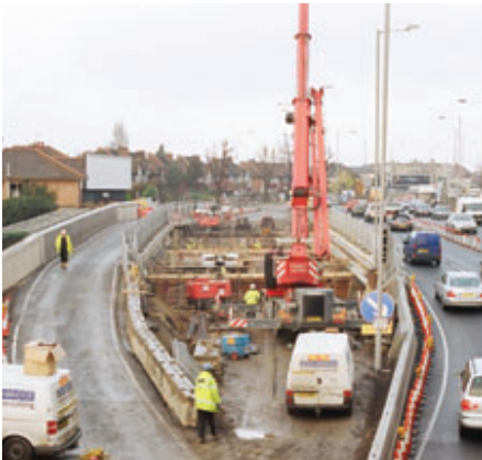
Perryn Road Bridge works
