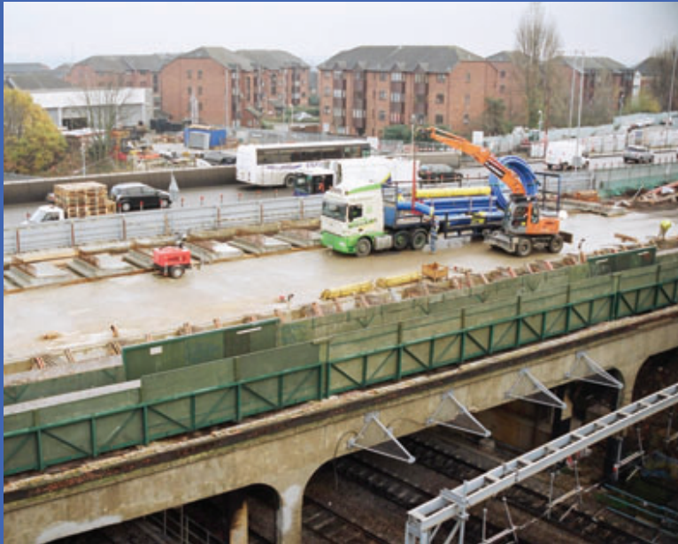
New bridge deck construction at Wales Farm Road Bridge
